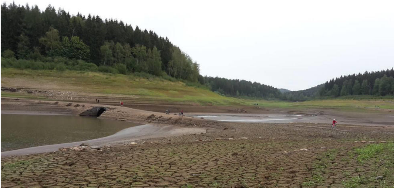
Fig. 3: The heavily lowered dam Lehmühle, picture: Petra Walther
