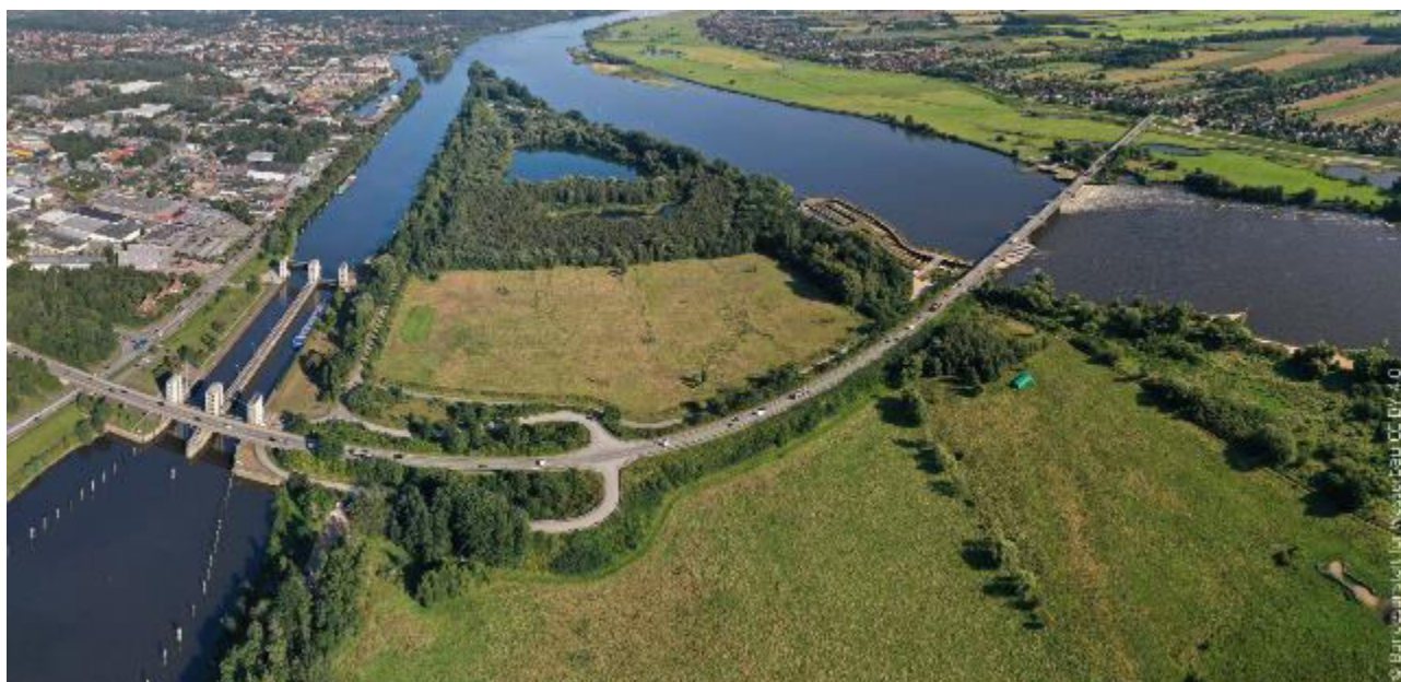
Fig. 1: A weir with sedimentation basin serves as a fictitious measure for the socio-economic study. The structure could be similar to the weir and its sluices in Geesthacht, lock canal with double chamber on the left, weir with four weir gates and fish ladder on the right, here aerial photo (Bundesanstalt für Wasserbau)
