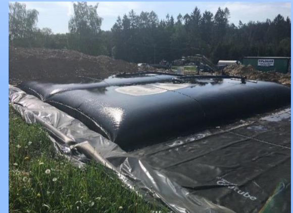
pump dredger + bags
