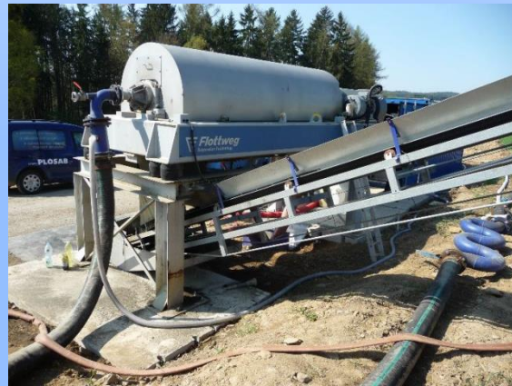
pump dredger + centrifuge
