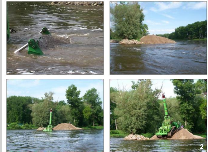
Dredging in the Czech Elbe, use of the underwater bulldozer "Komatsu"
