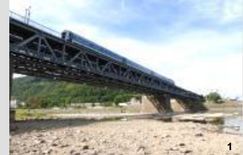
Railway bridge in Ústí nad Labem
