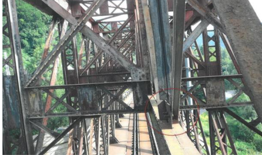
Railway bridge– original state
