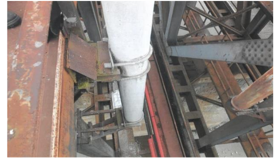
Railway bridge– original state
