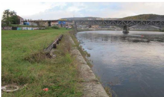
Left bank – before decontamination
