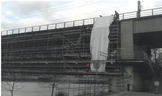
Railway bridge– during repair
