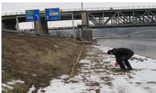
Left bank – after removal of contaminated soil, final sampling
