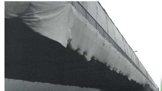
Railway bridge– during repair
