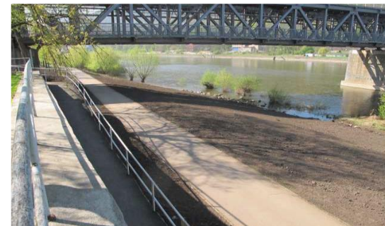
Left bank – after decontamination
