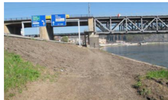
Left bank – after decontamination
