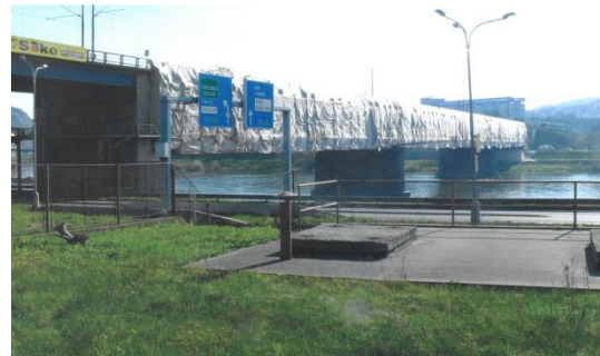
Railway bridge– during repair
