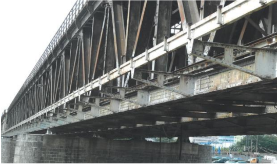
Railway bridge– original state
