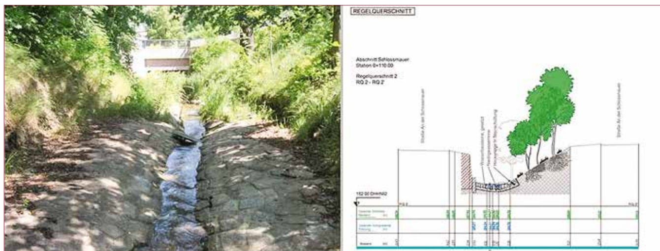
Fig. 1: Left: Outline situation in urban areas. Watercourse of the Mortelbach within Waldheim modified by concrete bed and bank stabilisation. These sections are subjected to a potentially significant flood risk (source: Landesamt für Umwelt, Landwirtschaft und Geologie), right: construction plan for hydromorphological mitigation measures of the Mortelbach considering the high demands of flood protection (source: Stowasserplan GmbH & Co. KG)
