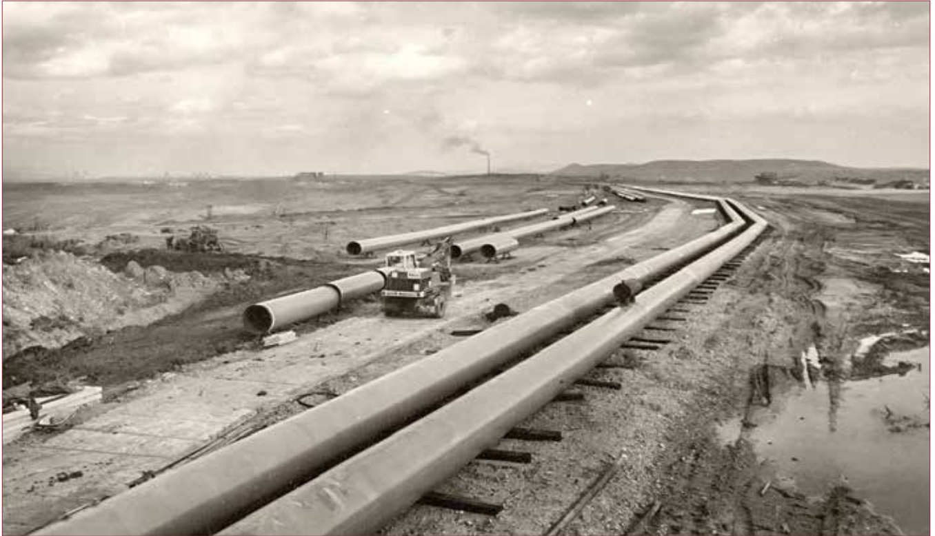
Fig. 1: View of Bilina in the Ervěnice Corridor in the direction of the town of Most – construction of the EC in 1981
