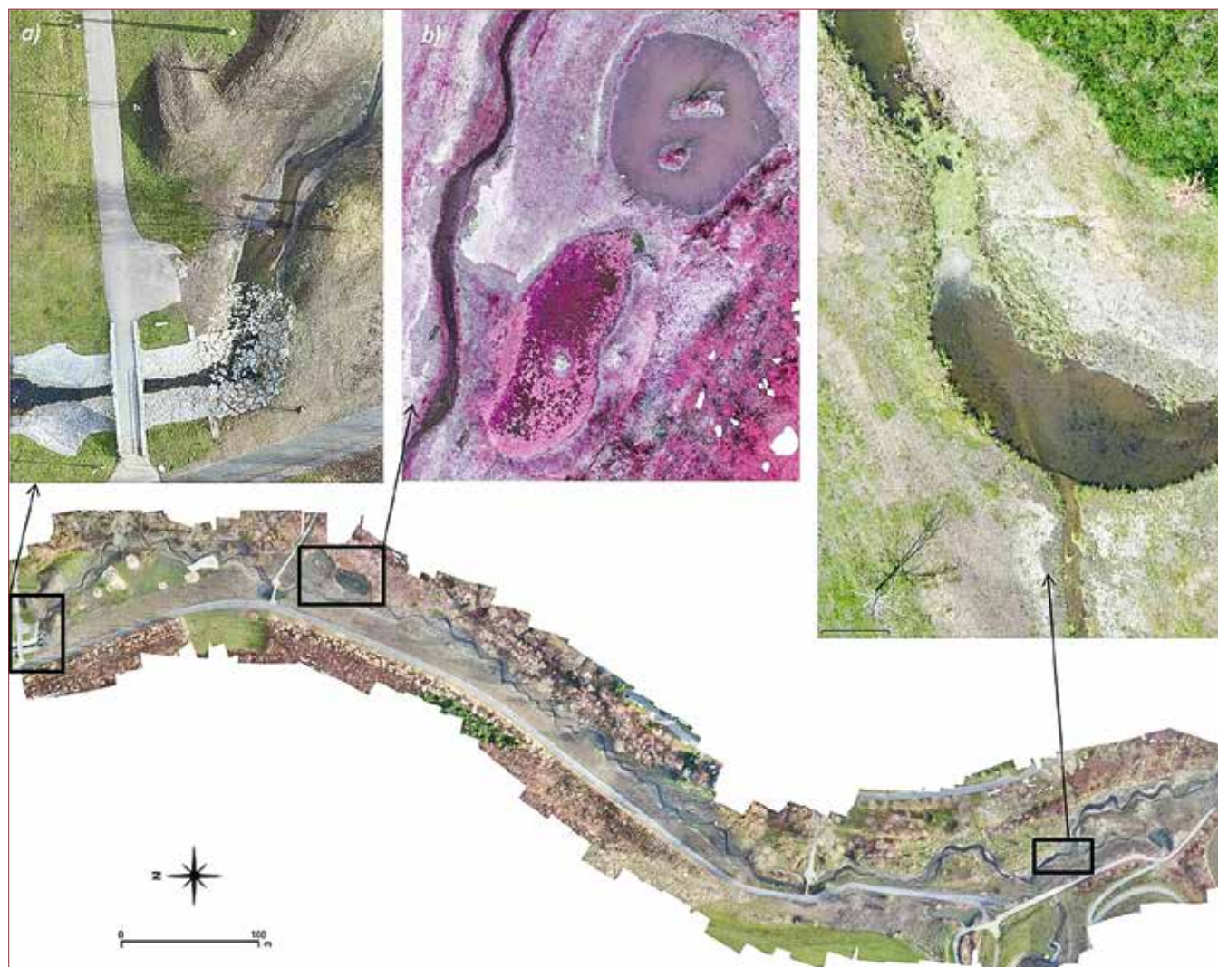
Fig. 2: Example of the potential of UAV orthoimage data for identification of stream properties and structures in the Hostavický brook, Prague. a) stream restoration works on the channel, b) identification of eutrophication at artificial ponds, created during the stream restoration, c) identification of the in-stream obstacle, resulting from wood debris after a spring storm. Data: Charles University in Prague, 2016.
