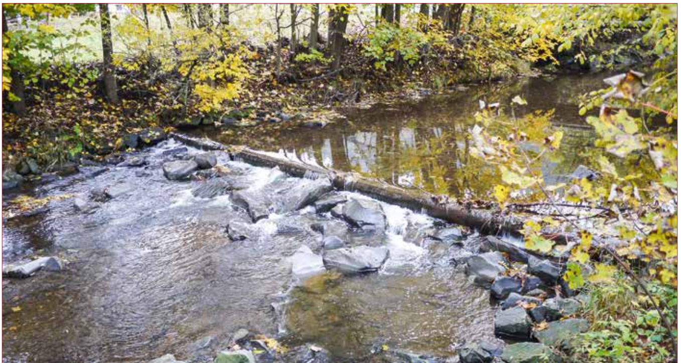
Fig. 2: Relatively low structures with not appropriate construction can create a migration barrier, mainly during low flow conditions.
